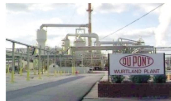
DuPont's Wurtland, Ky. plant produces a number of the building-block chemicals utilized in many consumer and industrial products. Here the operating tower is pictured visible from the center rear.
