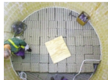
The FLEXERAMIC® ceramic structured packing is installed.
