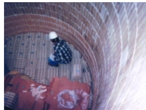
In order to optimize pressure drop reduction during a recent expansion, Marsulex opted for Koch's FLEXERAMIC structured tower packing.
